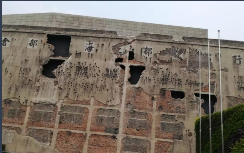
One side of the Sihang warehouse. Original.
